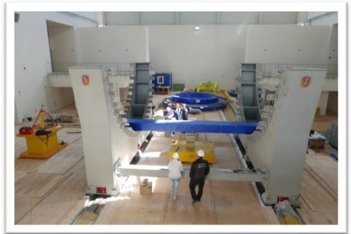
The first iron yoke beam is installed
